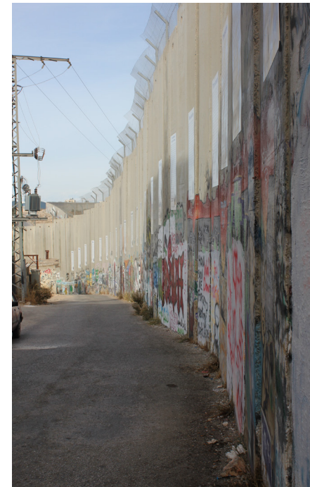
In urban areas like this, the wall takes the form of an eight meter high concrete barrier.
